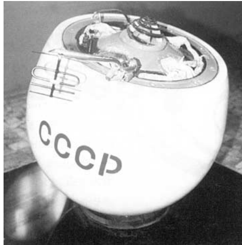
Figure 14. The Venera 4 probe, about one meter in diameter and weighing 383 kg.
